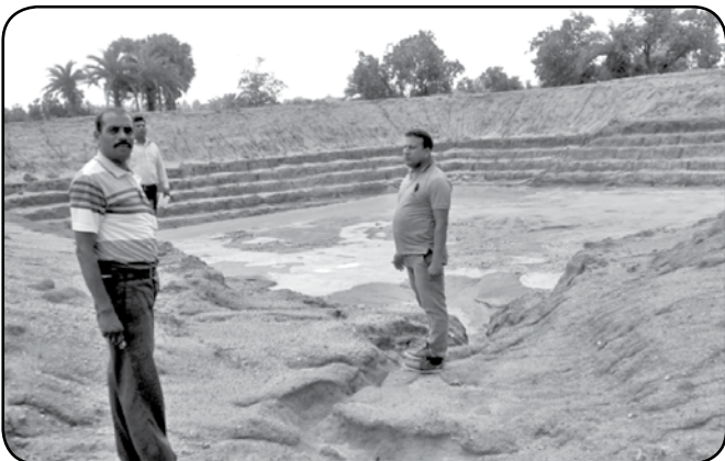
Water Conservation structure
